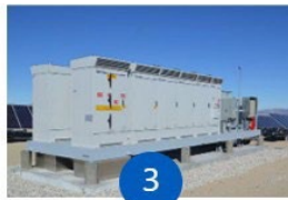
Inverter/transformer skid
