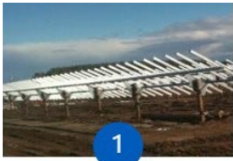
Racking mounted on piles
